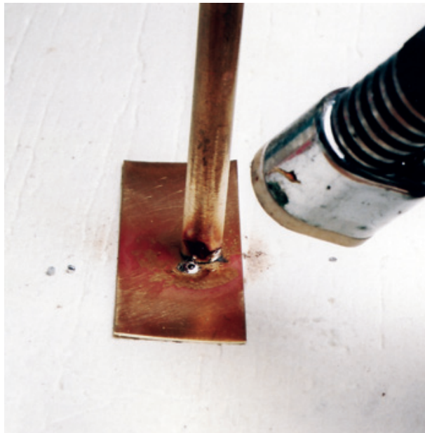
Figure 10.19: In this view, you can see how the heat has started to melt the solder balls.
