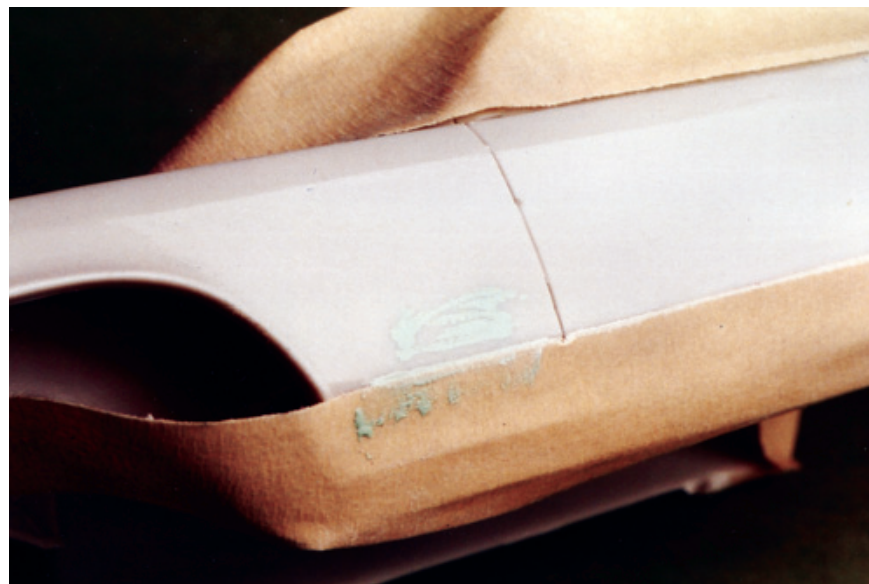
Figure 9.9: Tape off the area around the spot to protect the surrounding area from excess putty, greatly reducing your work. Mix a small amount of catalyzed putty and fill in the area, extending the putty just a bit beyond the excavated area.
