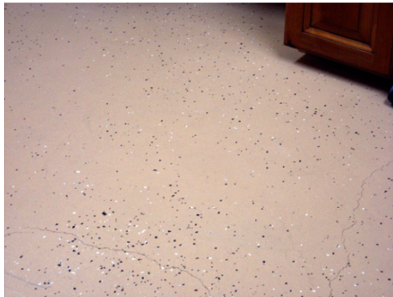
Figure 6.8: Coating your floor with an epoxy finish may seem like an extravagance, but it's a great idea. (Brian Dees' shop/photo)
