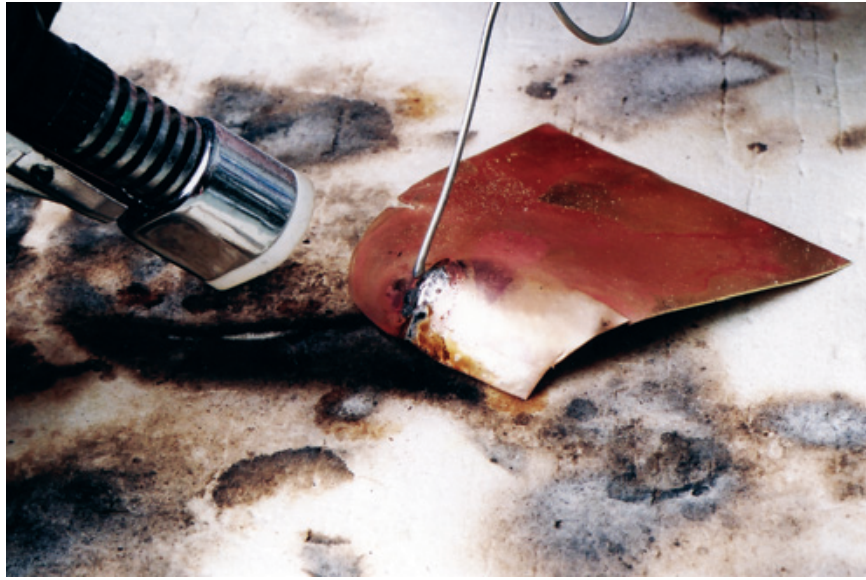
Figure 10.48: After fluxing the joint at the front of the hood, lightly heat up the panel and melt some silver-bearing solder into the joint. Don't use regular rosin-core or acid-core solder: neither are strong and both melt at too low a temperature. Once the solder has flowed into the joint, lightly play the flame over the area to help the solder flow along the joint. You'll need to experiment on this technique since you don't want the pressure of the flame to literally blow the solder out of the joint. Now, solder up the two cuts made at the side of the hood.
